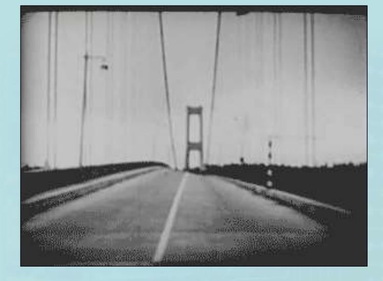
The Tacoma Narrows bridge collapsed due to torsion and shearing forces produced by the wind.
